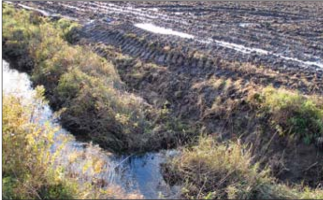
Photo 17: Failure caused by an excessive load Source: Mikael Guillou, MAPAQ
