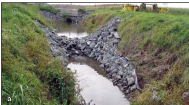
Photos 7 (a and b): Energy dissipating sill Source: Jacques Goulet and Victor Savoie, MAPAQ
