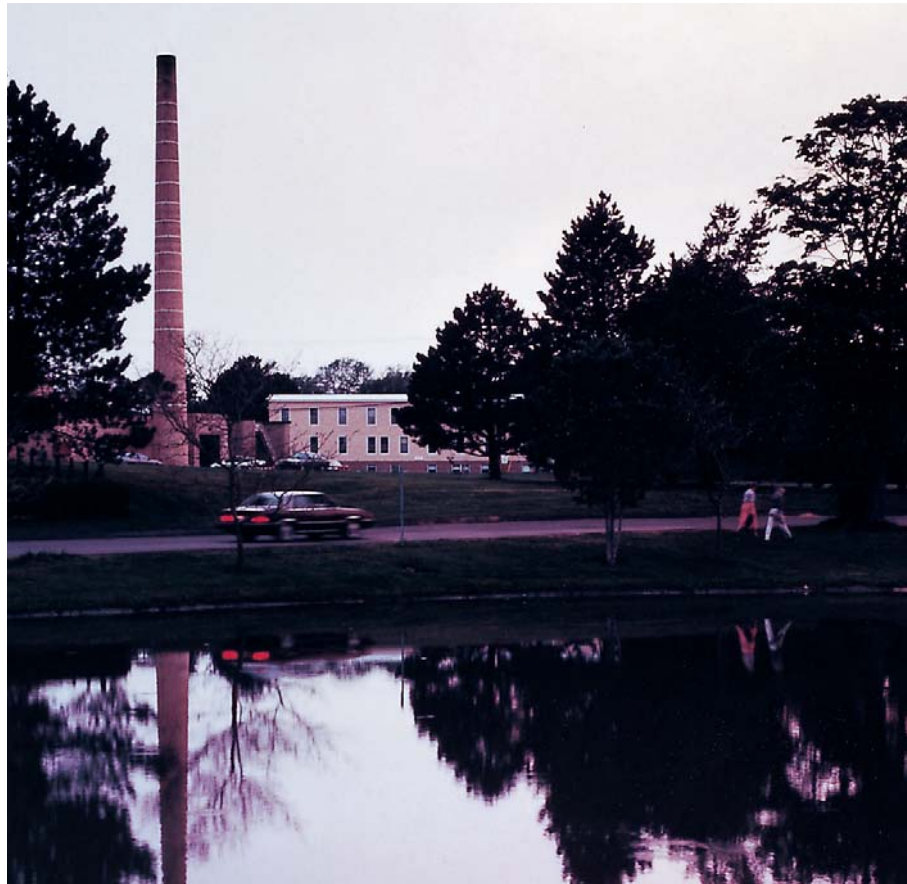
FIGURE 13 INSTALLATION DE CHAUDIÈRES DU PRINCE EDWARD HOME
