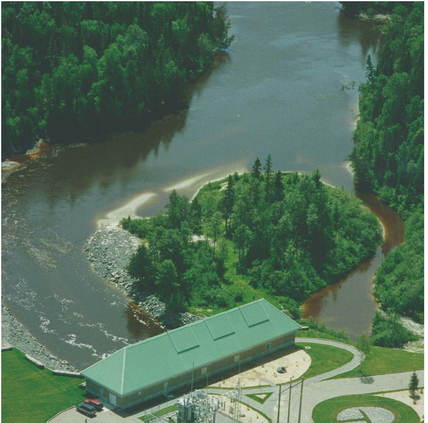
Centrale de Wawatay. Regional Power Inc.
