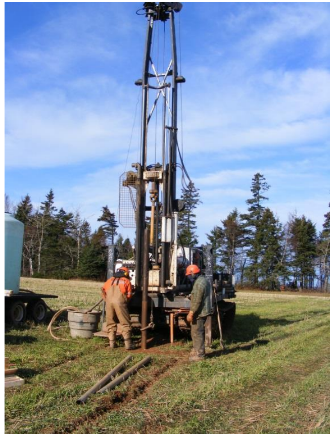
Drilling of groundwater monitoring wells at Harrington Farm (AAFC) in Prince Edward Island. Crédit photo : Serban Danielescu, Ph. D. AAC Canada
