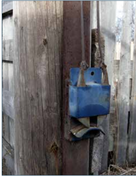
Figure 26. Example of a closing mechanism (latch)
