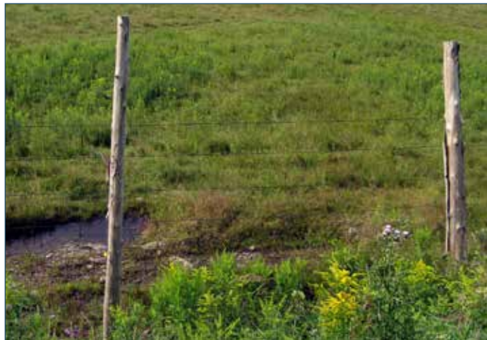
Figure 2. Example of a fence made with high-tension steel wire
