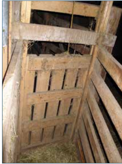
Figure 15. Example of a guillotine door
