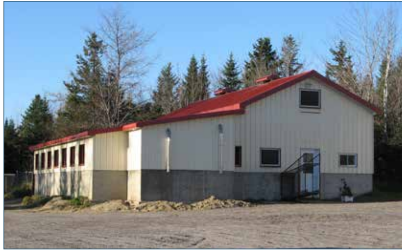
Figure 6. Cold farrowing barn
